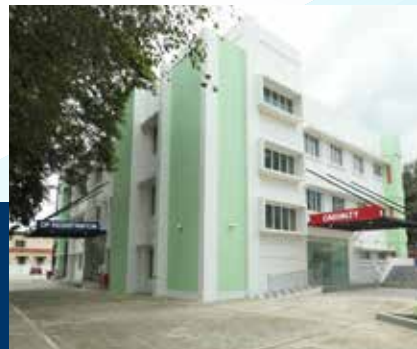
Taluk Hospital Ottappalam, Kerala
