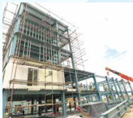
On-site steel Construction
