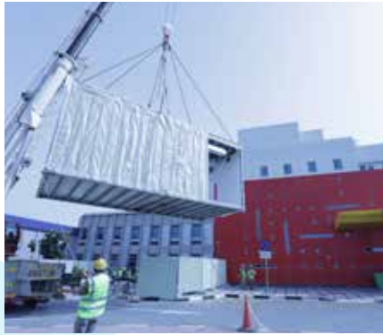
Modular Construction (PPVC)
