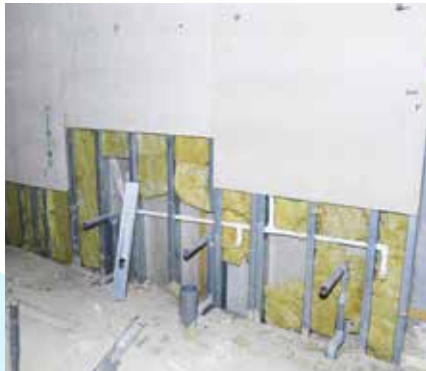
Cement Board Partitions
